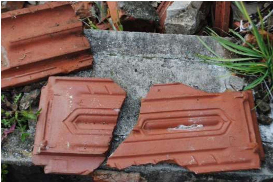
QBE3 – Broken clay roof tile that was presumably used as the roof covering of the farmstead prior to demolition.
