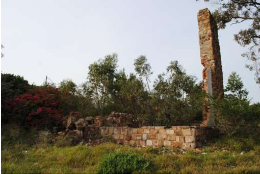
QBE3 - View taken from the approach pathway of the remains of the building. The stone plinth with partial stone chimney is visible. Widespread vegetation has established itself within the confines of the building footprint.
