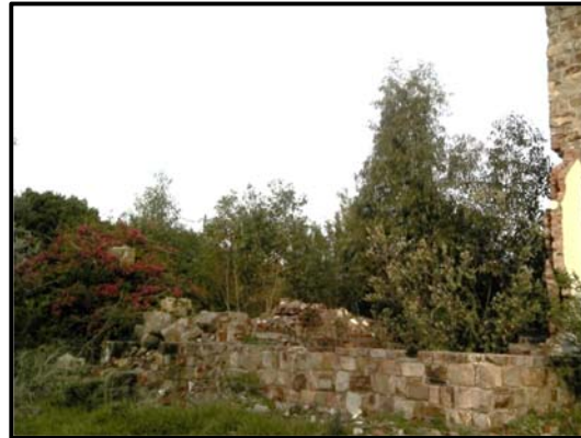
Ruins of a farmstead to the east of the site
