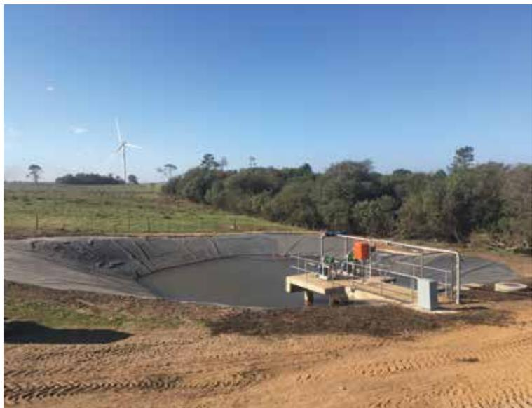
Wash water pond with recycling pump station.
