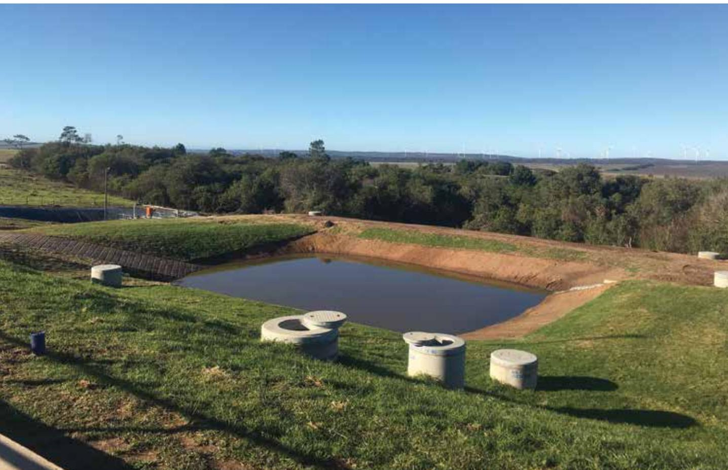
Secondary sludge pond with vehicle access and distribution manholes.
