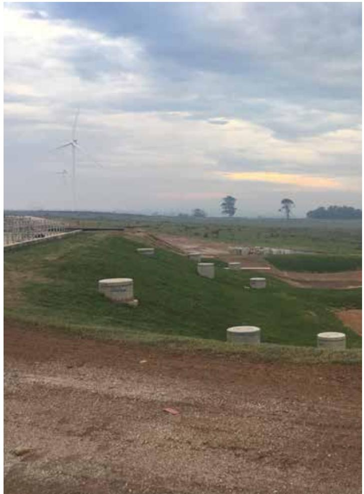
Sludge and wash water ponds prior to commissioning. Note rehabilitated slopes and embankments.
