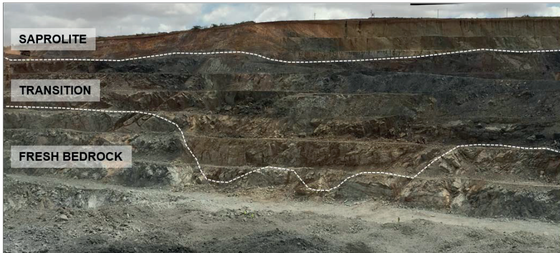
Figure 8: Weathered Rock Profiles across the West Wall, Essakane Pit
