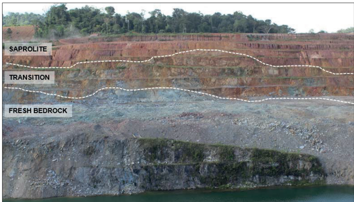
Figure 2: Weathered Rock Profile Exposed Through Bench Slopes at the Rosebel Mine, Suriname
