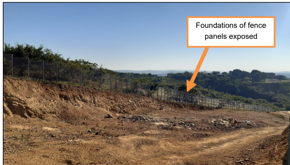
Plate 5: Exposed fence panel foundations (potentially undermined) and missing fences panels
