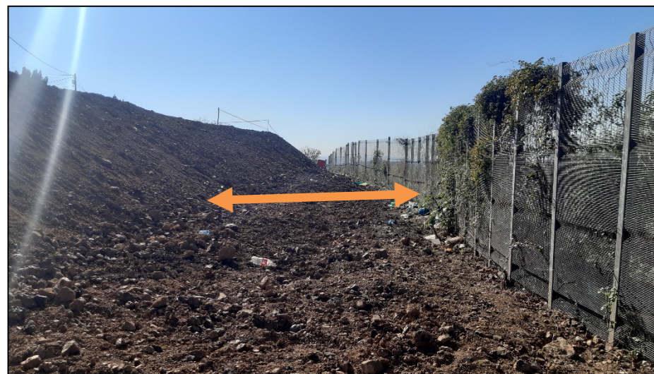
Plate 12: Toe of the transit camp platform pulled forward and out of the 5m forest buffer
