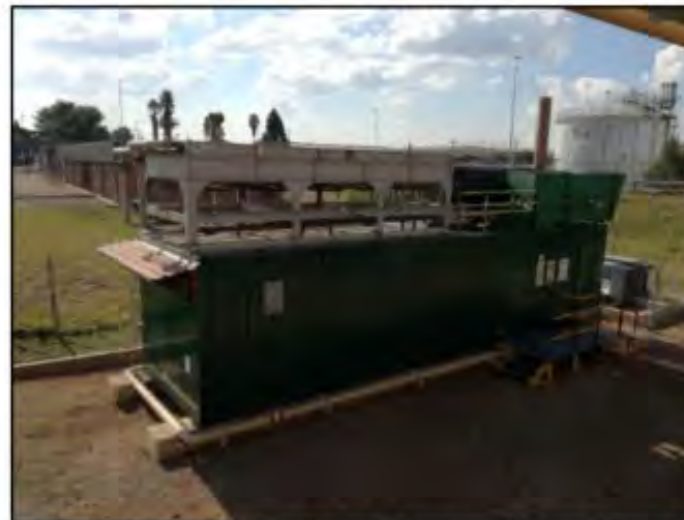
Figure 6-1 (b): Deutz containerised engine
