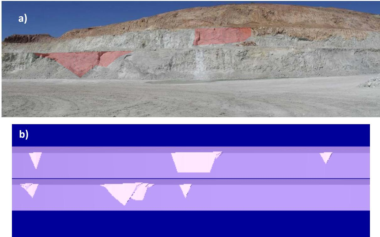
**Figure 8** Calibration on site of bench berm analysis. (a) Picture of the slopes benches in the southwest structural domain. b) Output of SBlock program showing the failed blocks removed (red zones) for this sector using Southwest structural domain data shown in Table 1.
