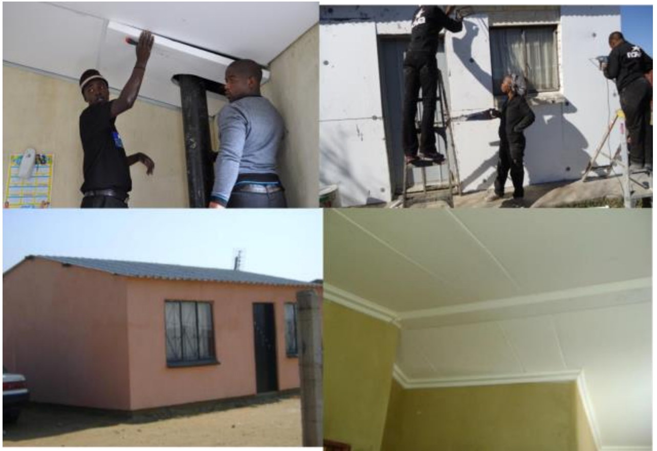
Figure B4 – insulation implementation in KwaDela, clockwise from top left: installation of ceilings requires precision and fit-for-purpose solutions for chimneys; attaching insulation to exterior walls; completed ceiling; completed exterior insulation, covered in pigmented plaster in the colour selected by the household
