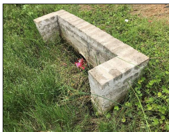
Plate 4-5: Existing culvert crossing within the CVB wetland confining flow
