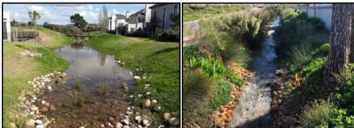
Plate 13-4: Examples of open swales, considered to be SuDs utilised for conveyance of stormwater
