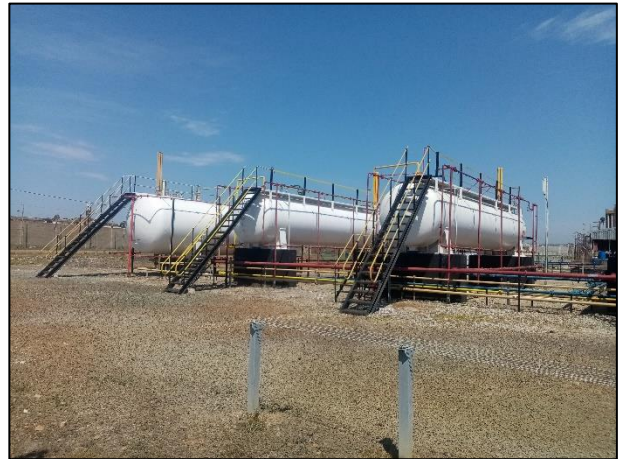
Photograph 12: Existing 45 and 90 m 3 LPG storage tanks on the site
