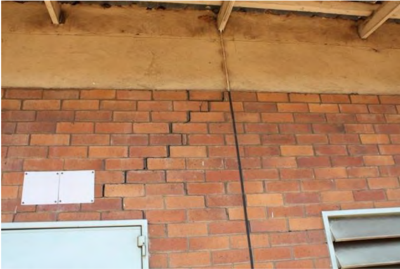
Figure 11: Example of blast induced damage.
