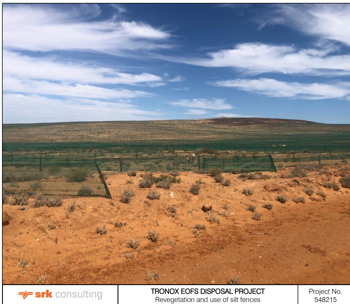
Figure 4-5: Photo showing revegetation in processes with fences to trap windblown soil and prevent soil between the fences from being blown away
