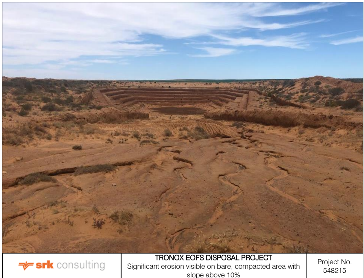
Figure 4-2: Photo showing significant erosion visible on a bare, compacted area with a slope above 10%
