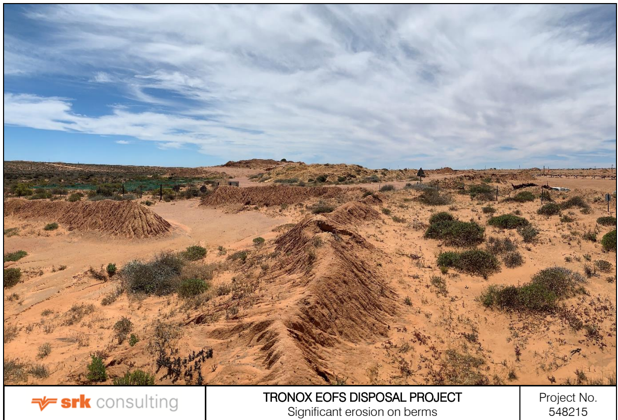
Figure 4-4: Photo showing significant erosion on berms
