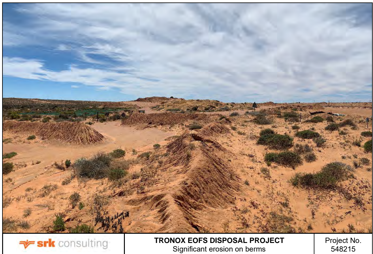
Figure 2-7: Photo showing significant erosion on berms
